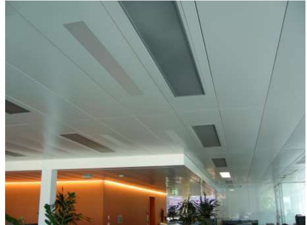
WK-D-PP in Metalldeckenplatte
