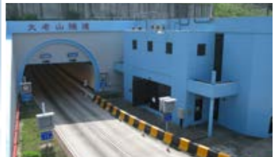
Tate's Cairn Tunnel, Hongkong
